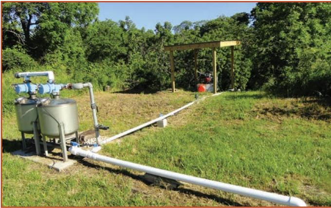
Figure 7. A sand filter (foreground) filters creek water delivered with a gas-powered pump (background).
